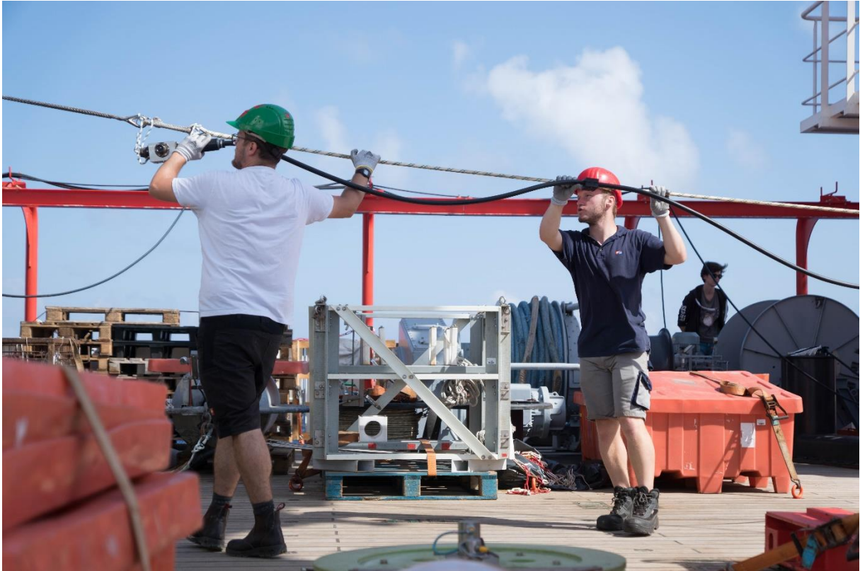
Michel Kühn and Florian Petersen during the recovery of the P-Cable making sure the cross-cable drums up properly on the winch. Photographer: Jonas Liebsch.
